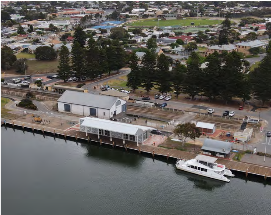
A German-style café and restaurant has been approved for the commercial portion of the newly rebuilt Goolwa Wharf Shed.
