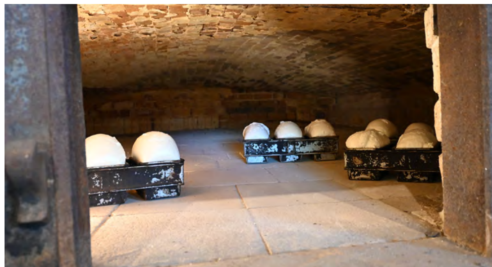
The oven of the former bakery would take three to four days to heat up.
